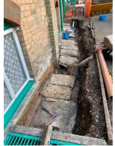
Excavation in the car park, credit Bruce Longstaff
